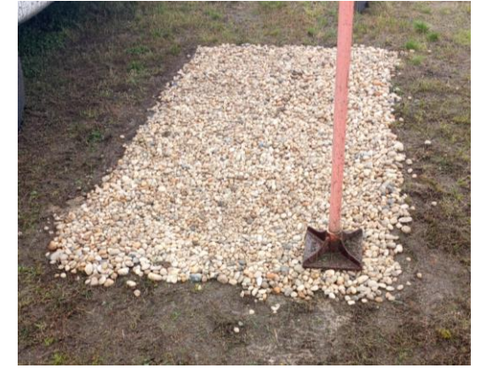
Tamp and level stone
