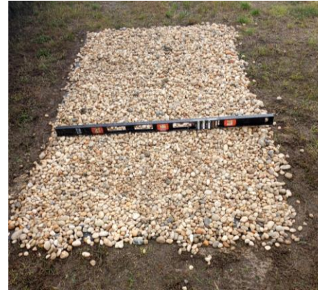
Layout six 50 lbs bags of stone and rake level
