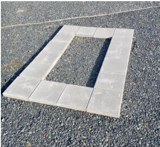
Arrange paver blocks in the pattern shown. Level blocks
