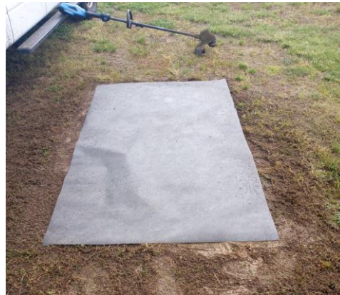
Once ground is bare lay down weed barrier cloth or tarp 4 foot by 8 foot
